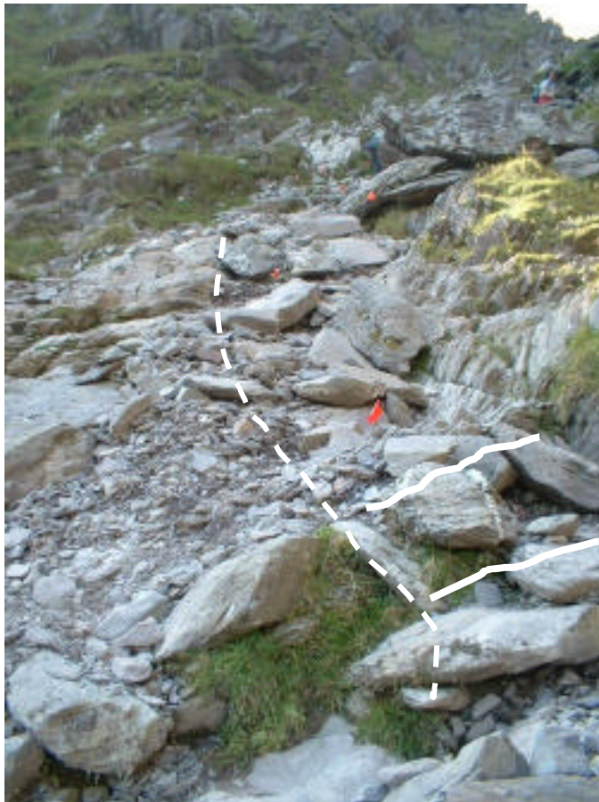
Figure 8. Well constructed rock steps at this type of location will improve route finding and assist soil stabilisation.
