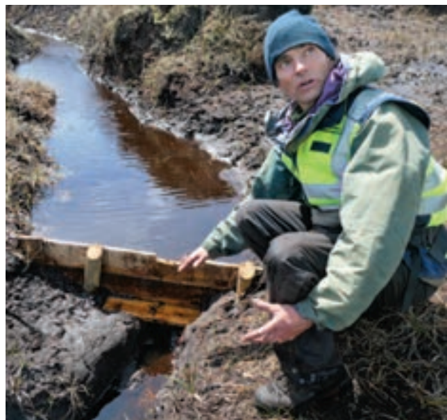
Hugh McLindon at a dam on Barnacullian, showing how these 'leaky' dams slow the water flow and help re-wet the bog. Sphagnum mosses will be added to these pools to hold water and enable carbon capture.
