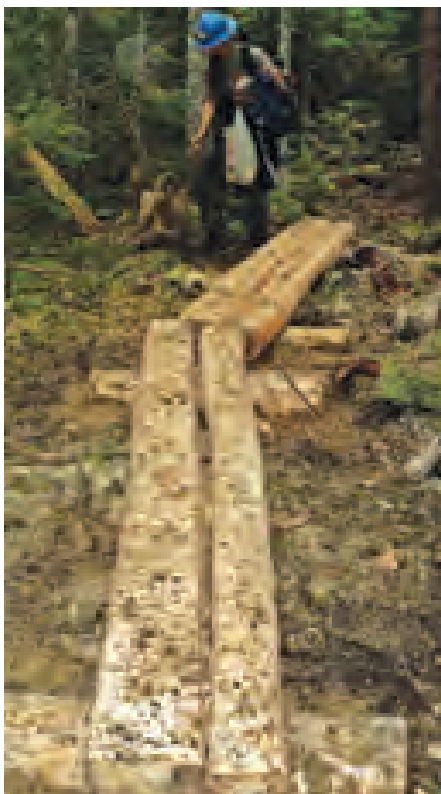
Bog bridge built on site using local cedar trees.
