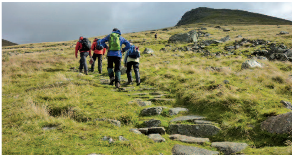
Stone-pitching on Helvellyn in the Lake District, a mixture of aesthetics and engineering, with all work done by hand. This path carries approximately 100,000 people each year.
