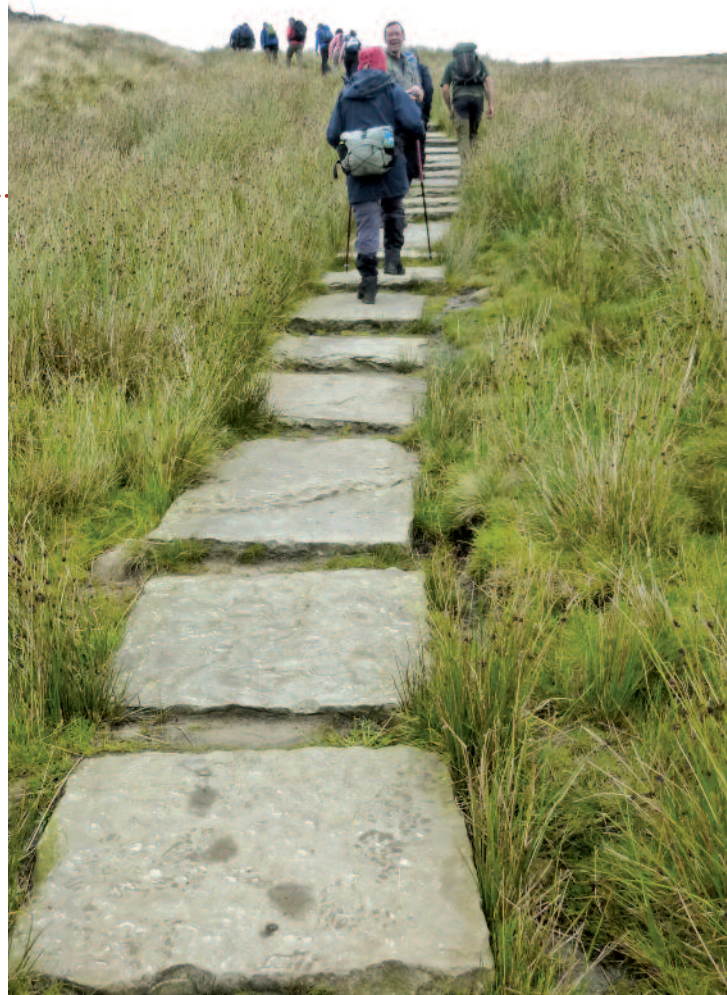
Flagstone path on Pen-y-Ghent in the Yorkshire Dales National Park. Large flagstones don't sink into the peat and they provide a durable path surface which allows re-growth of the vegetation on either side.
