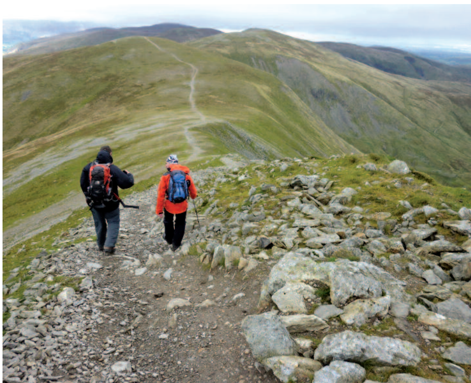
Descending from Helvellyn Lower Man, walking towards White Side. Erosion has been controlled here by placing stones and re-seeding on the right-hand side of the path to contain people on a narrower line.
