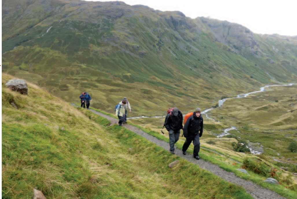
Reversal path below Stake Pass in the Borrowdale areas of the Lake District; created by removing the organic soil layer and mounding up mineral soil to give a firm path surface with a drain alongside.
