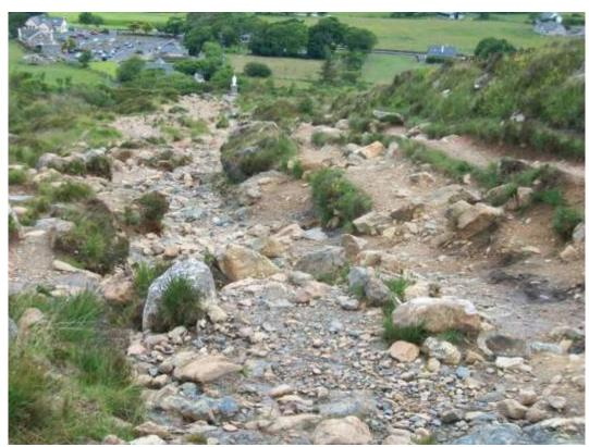
Section 1 – Looking northwards down the path to the start – braiding and turf "islands" very apparent, as is lack of any drainage. During heavy rain this would resemble a stream.
