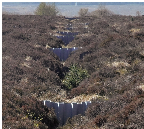
Plastic piling can be used to block ditches and restore bogs
